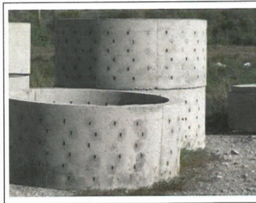
Figure E.4. Dry Well #1 – Structural Prefabricated Chamber.
